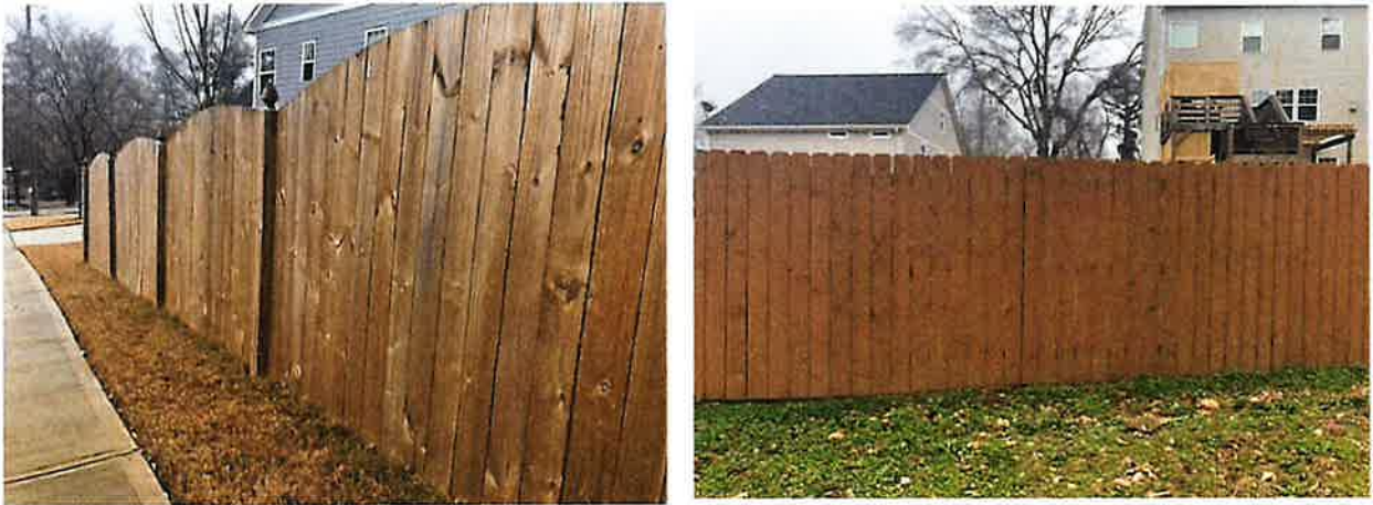
Examples of the finished side of a fence
