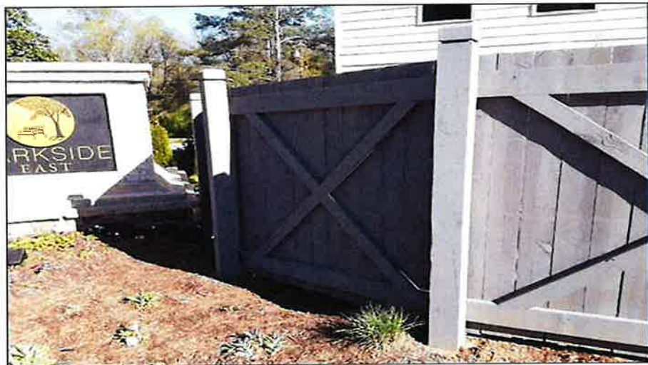
Dual sided fence with decorative elements
